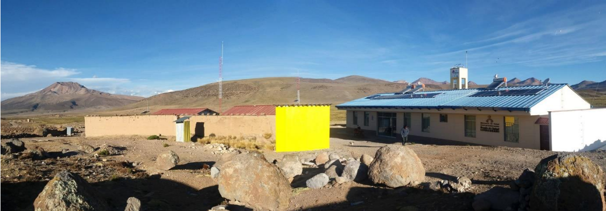
Picture 1: Coracorani Health Centre - water contaminated by volcanic activity is treated using a small drinking water treatment plant.
